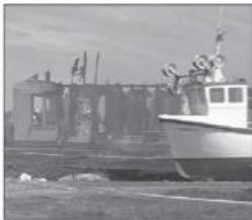
The charred remains of Judith and Geoffrey Johnson's home. Photo: Shetland Times
